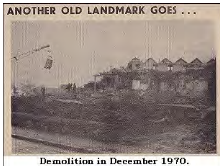
Demolition in December 1970.
