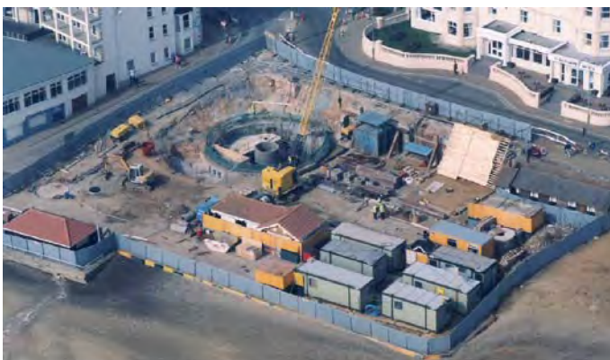
Extensive alterations taking place in March 2000.
