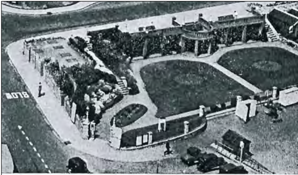
Final layout of the Gardens prior to the bandstand being built.
