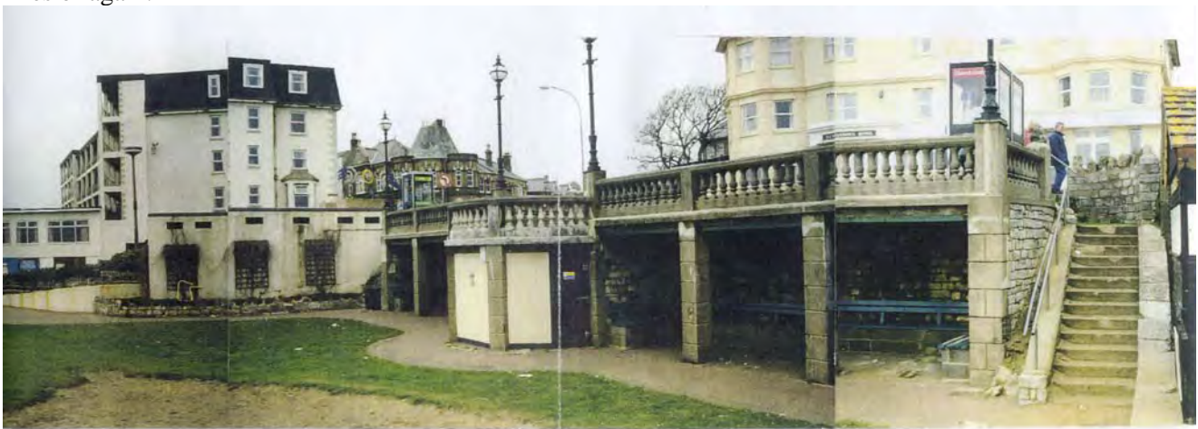
One of the last pictures taken of the Gardens prior to demolition, circa 1999.
