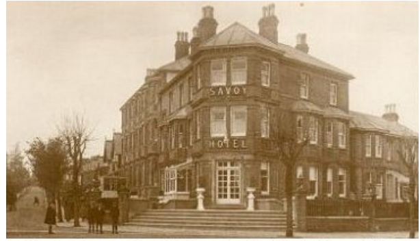
The newly constructed steps leading to the Lounge Bar and eventually the way to the Dive Bar.
